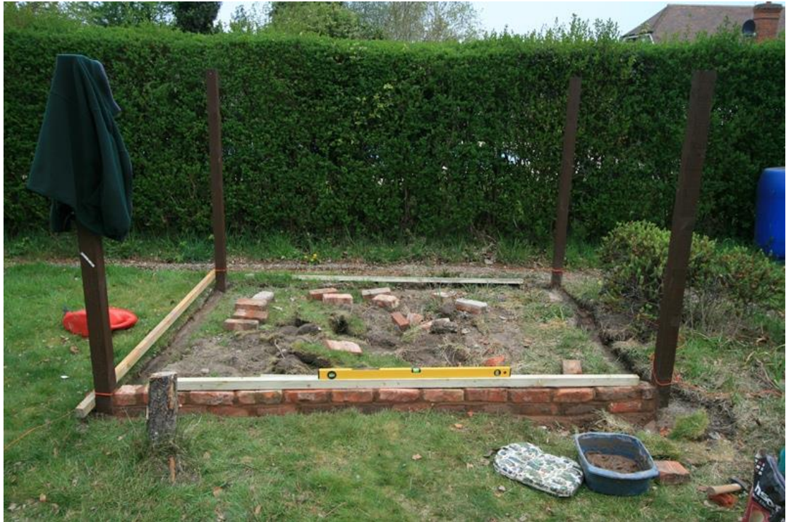
Figure 13 – Laying the two levels of brick
