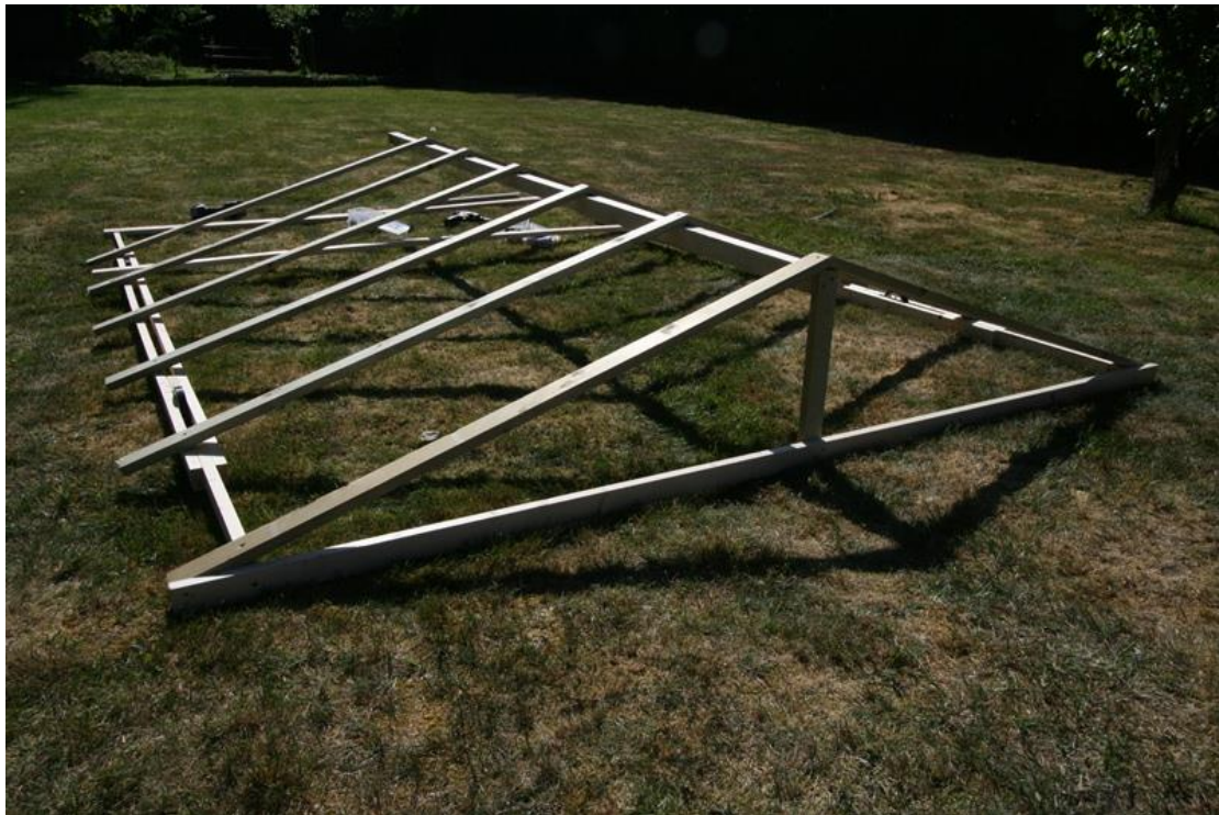
Figure 31 – The (nearly) completed roof frame
