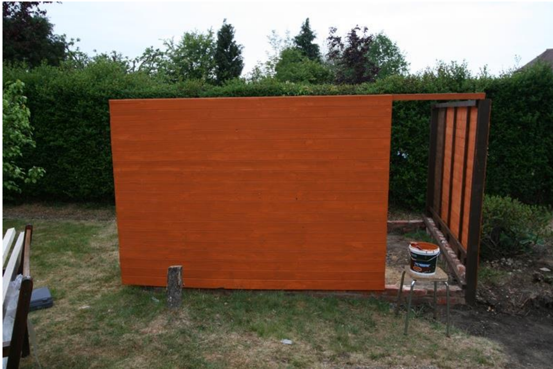
Figure 25 – Front complete with gap for door
