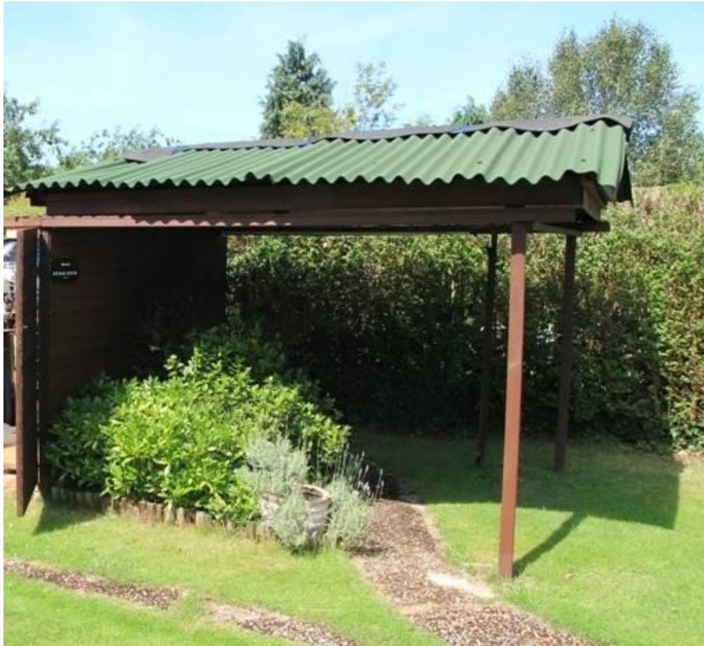
Figure 45 – Roof runners and supports completed
