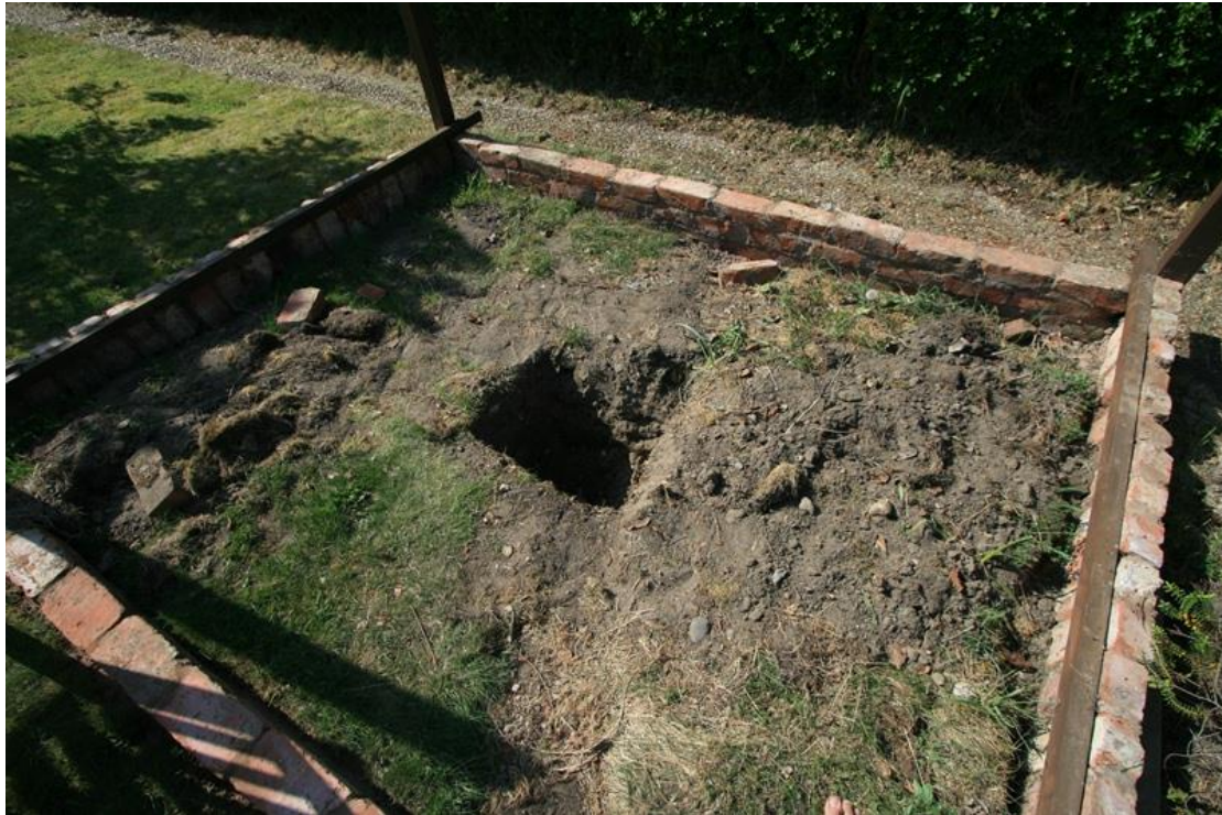
Figure 15 – Brick base completed (hole for the pier concrete base also visible)
