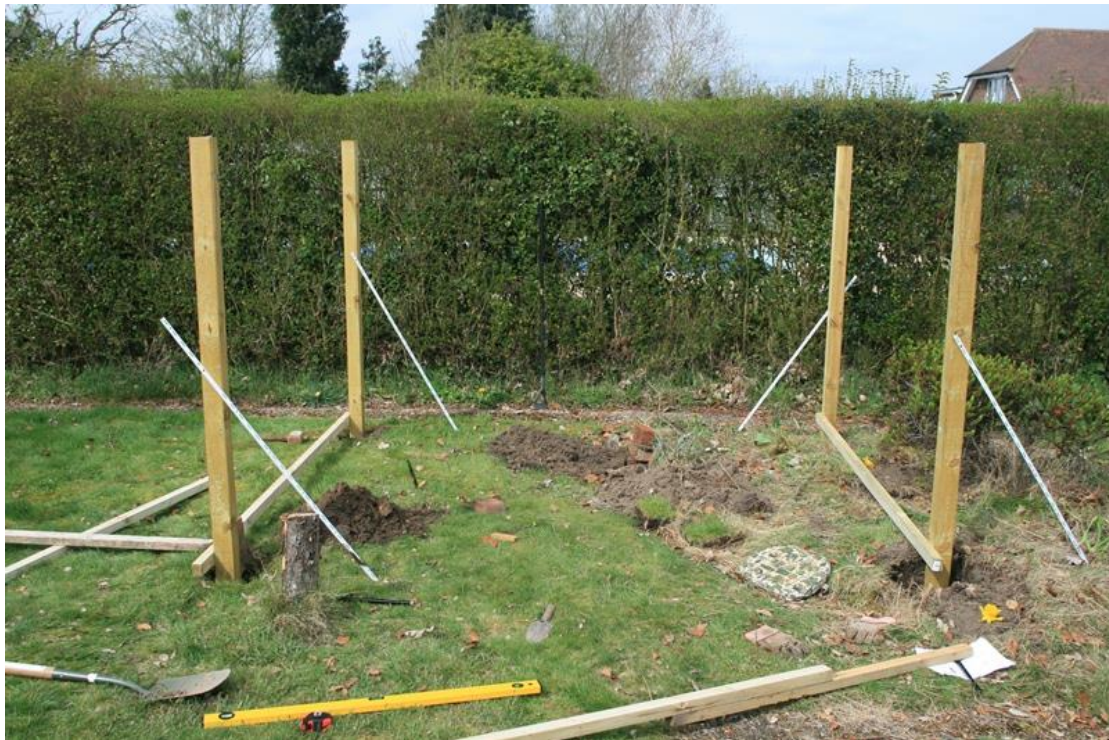
Figure 8 – Ensure the corner posts are correctly spaced, level and square to each other
