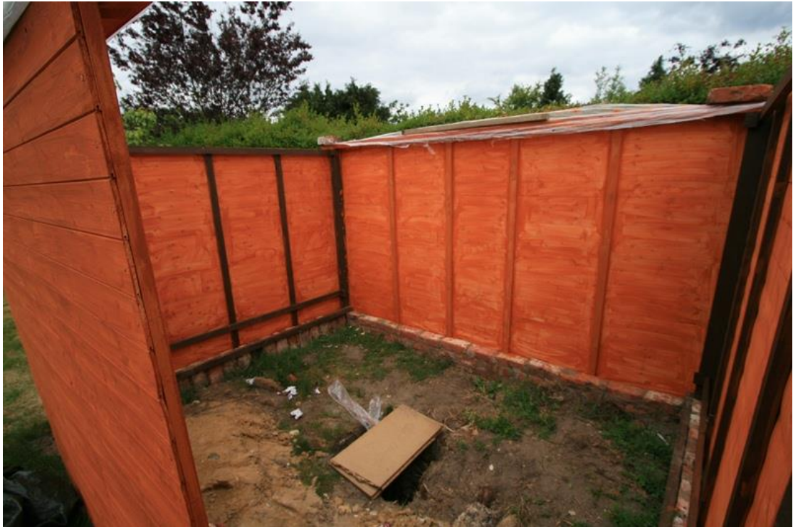
Figure 29 – All sides complete – view through door
