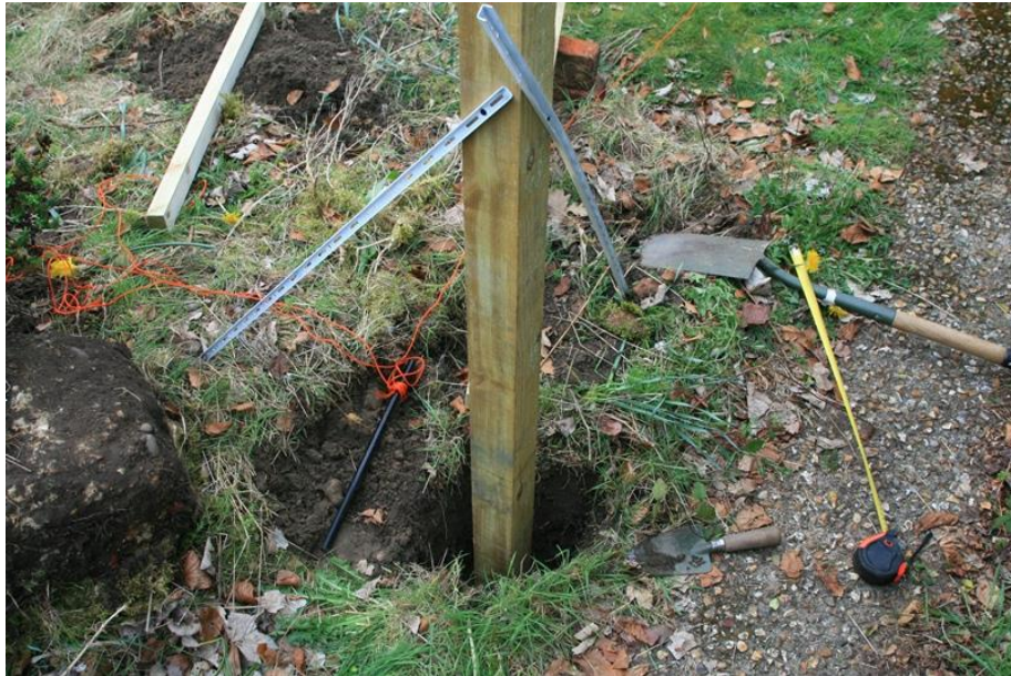
Figure 5 – Dig in the first corner post (temporary supports also visible)
