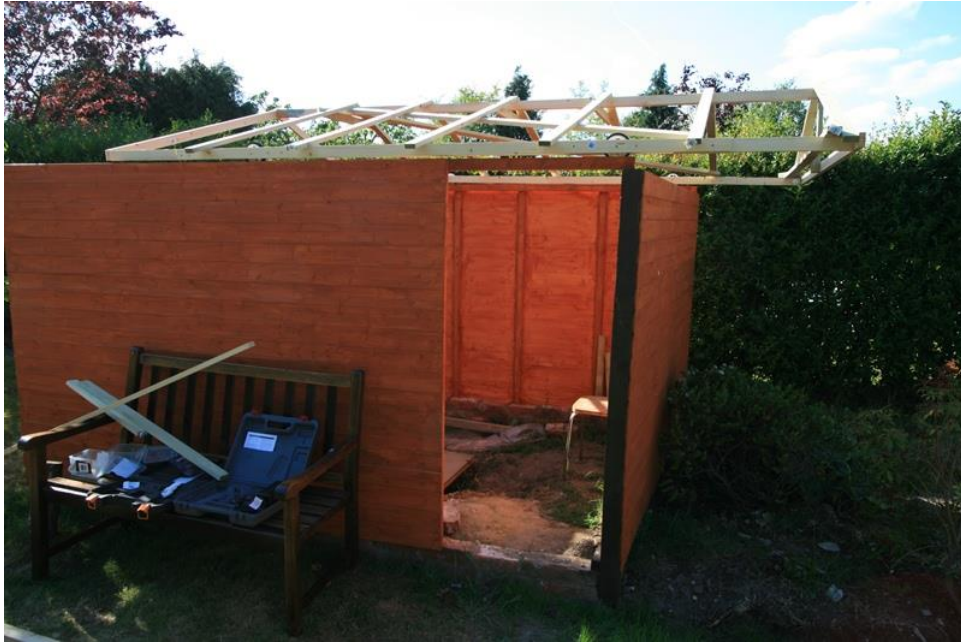
Figure 34 – Check that roof moves freely before adding bitumen sheets
