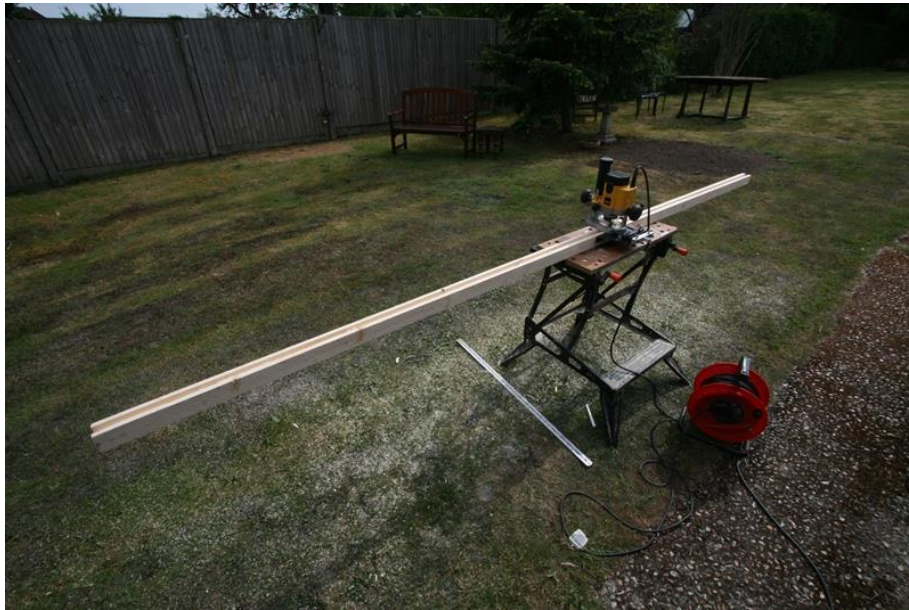
Figure 21- Start making the roof runner
