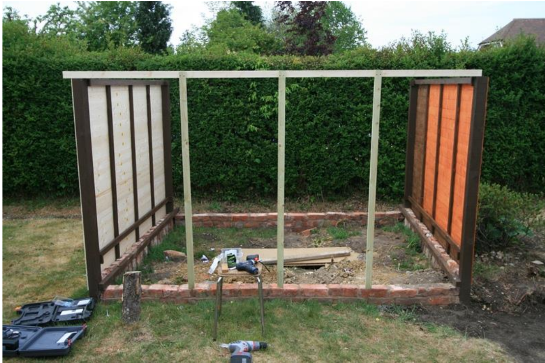
Figure 23 – The first Roof runner in place and the second side
