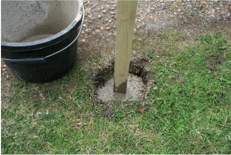
Figure 44 – Roof runner supports posts concreted into ground
