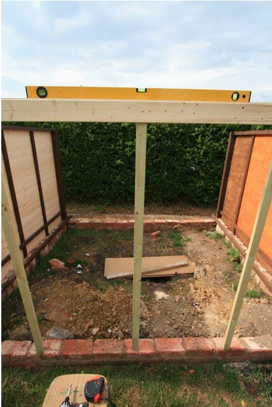
Figure 24 – Ensure roof runner is level
