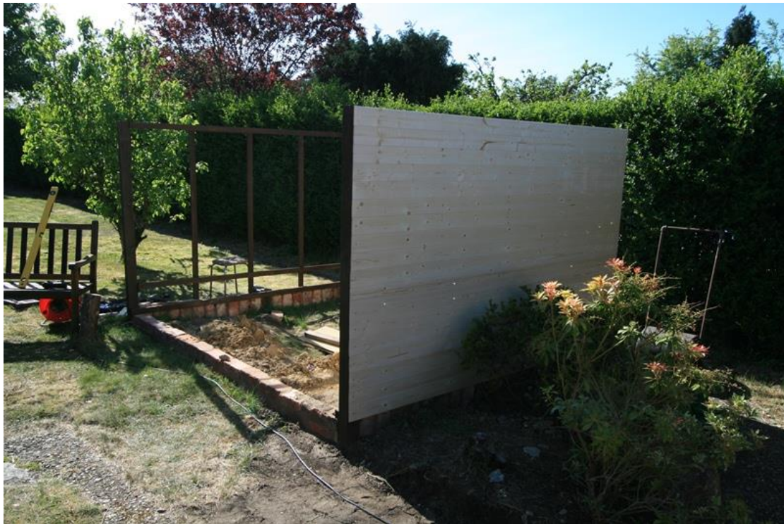
Figure 18 – Screw Shiplap cladding to the frame
