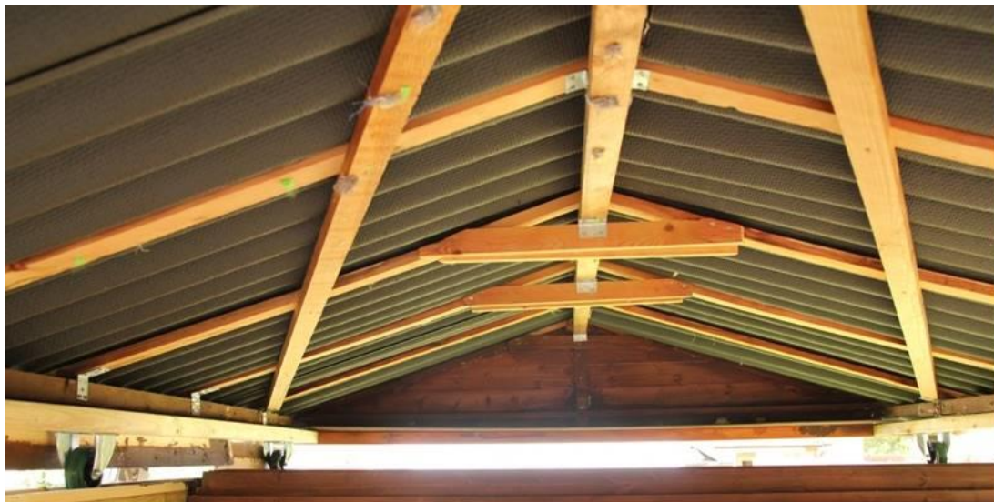
Figure 35 – Final roof assembly in place – note metal brackets at every joint
