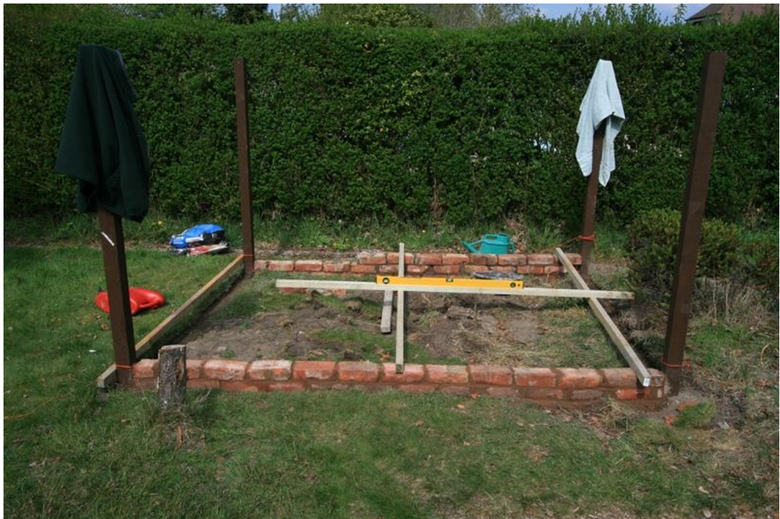
Figure 14 – Checking everything is square and level
