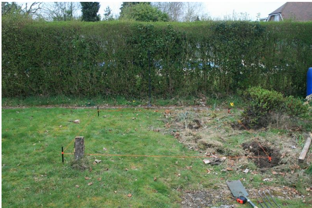
Figure 4 – Cleared the ground and marked out observatory area
