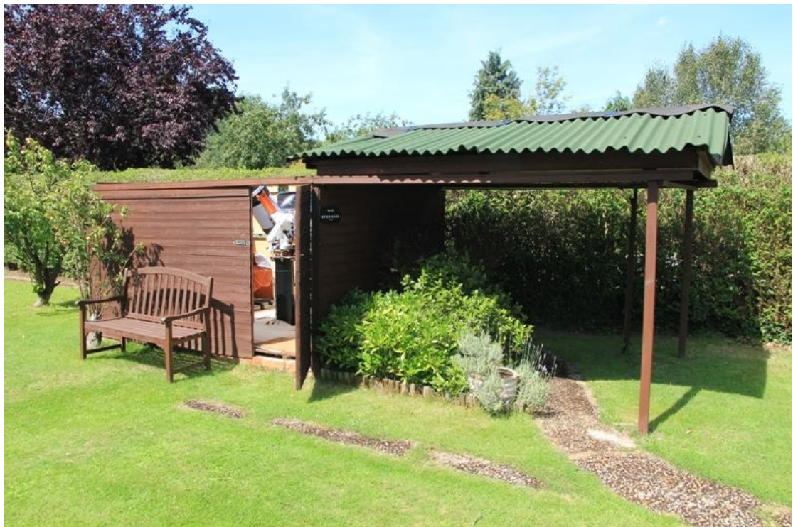
Figure 38 – Roof completed and retracted
