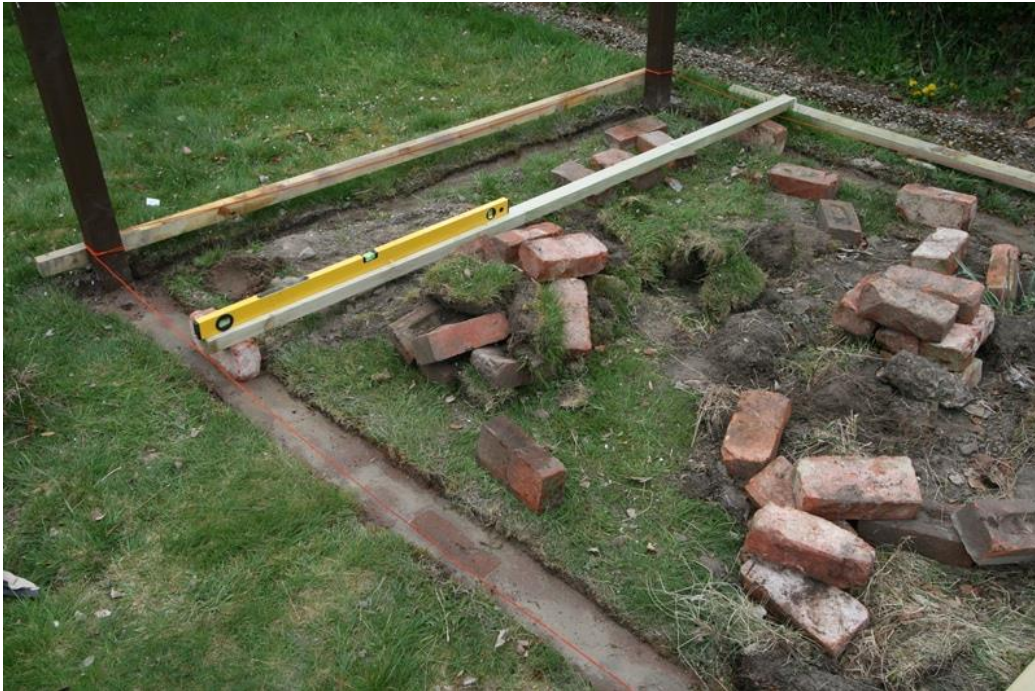
Figure 11 – Foundation done - make certain it is square and level
