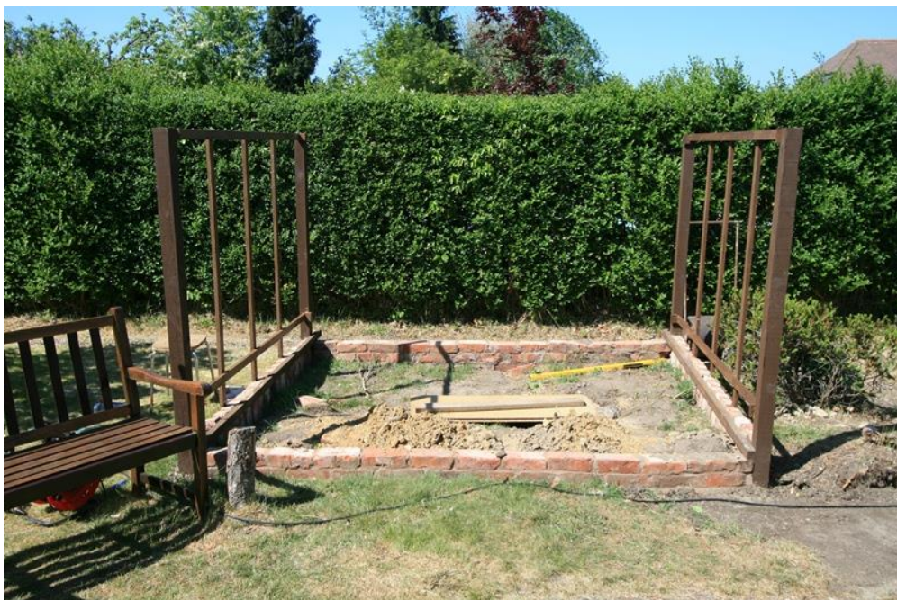
Figure 17 – Side Frames In Progress
