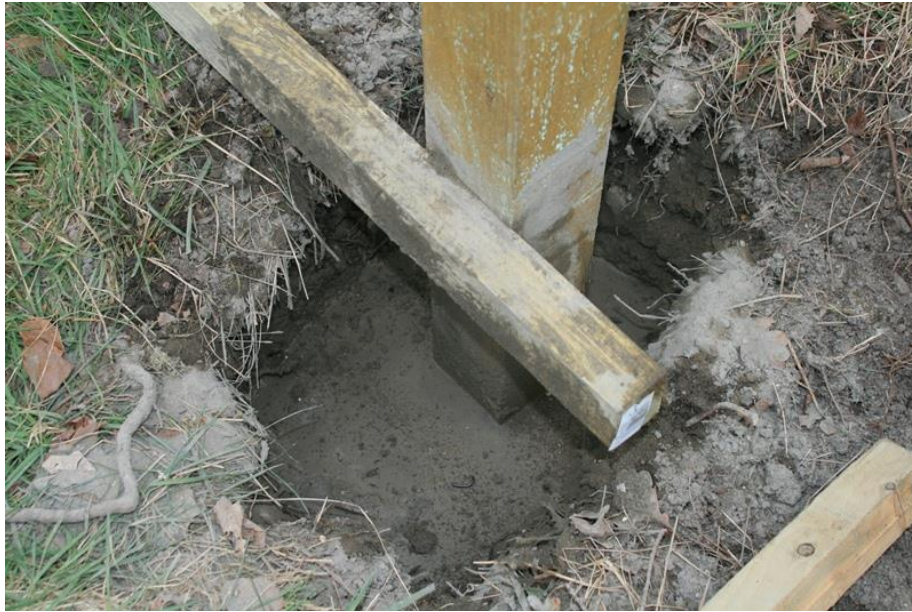
Figure 7 – Concrete each post (temporary cross support also visible)
