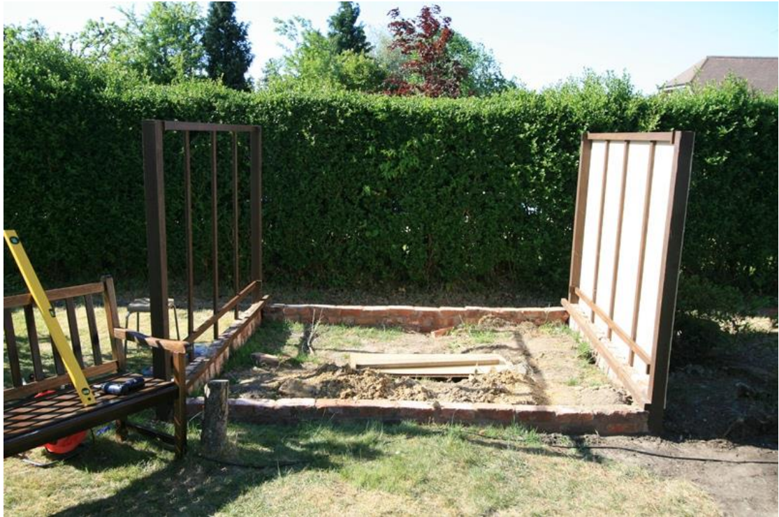
Figure 20- First side completed
