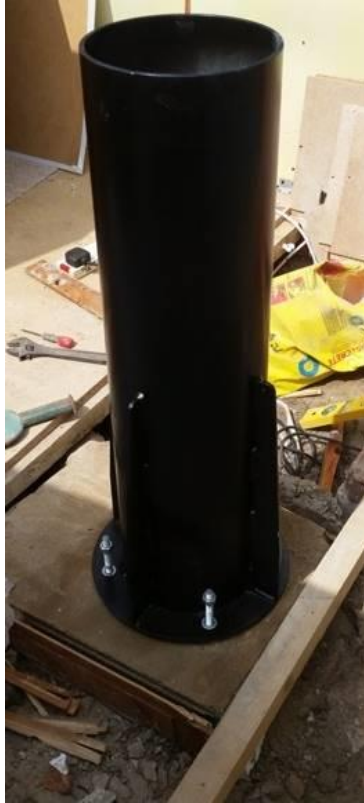
Figure 42 – Pier lowered onto the concreted in bolts
