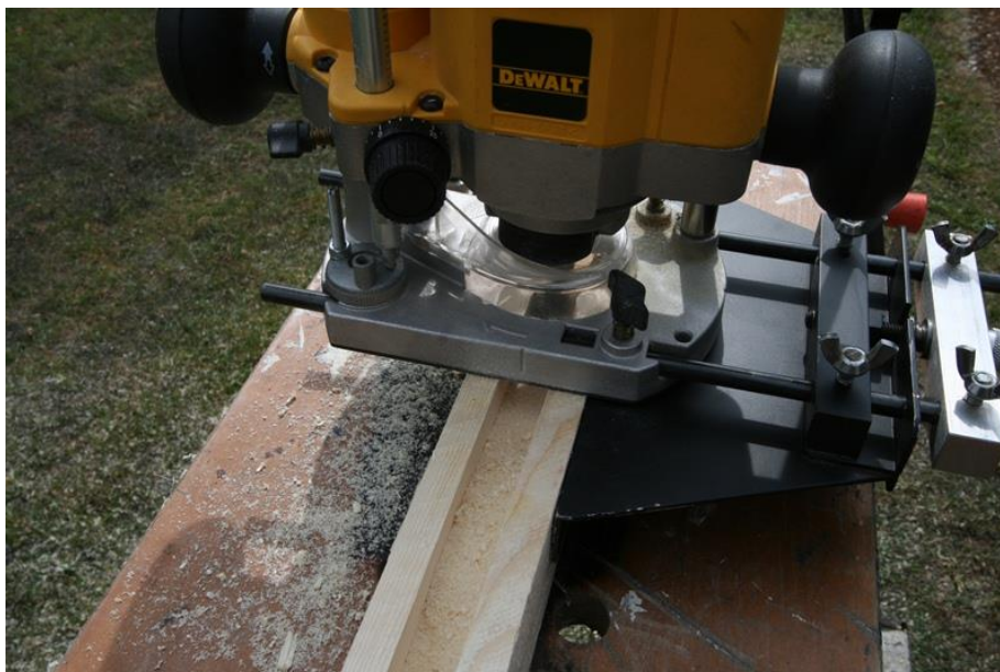
Figure 22 – Cutting out a channel for the roof wheels to run in
